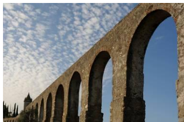
Roman Aqueduct in Evora
