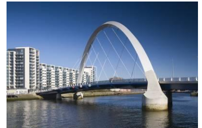
Clyde Arc Bridge
