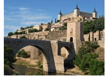
Bridge over Río Tajo
