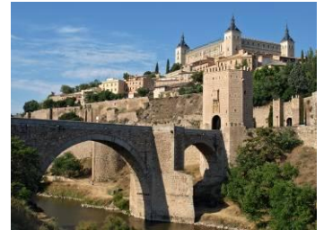
Bridge over Río Tajo
