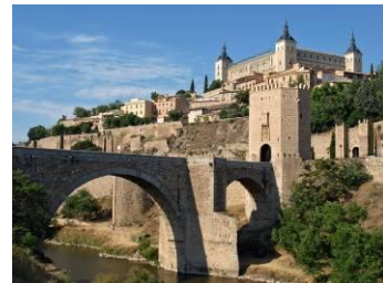
Bridge over Río Tajo
