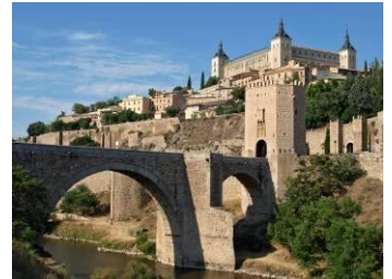
Bridge over Río Tajo
